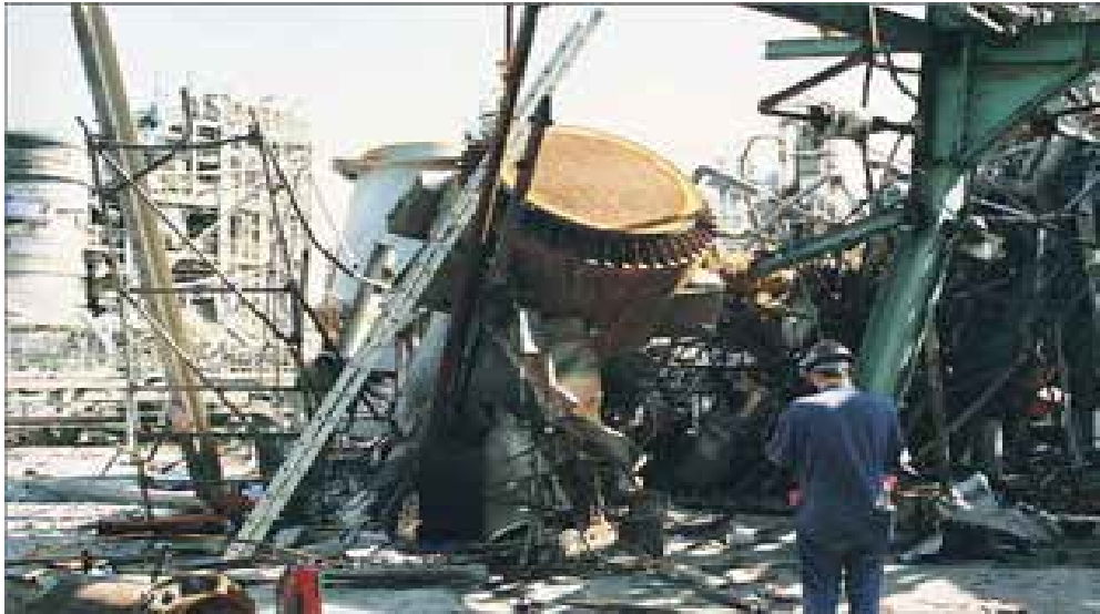
Figure 5.12 Ethylene Oxide Distillation Column Reboiler after Explosion
