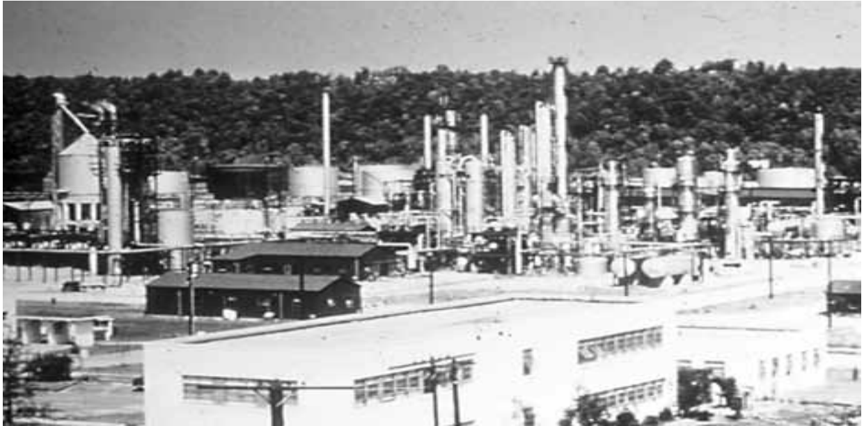
Figure 5.1 Older View of Plant Before Explosion Showing EO Tanks in Foreground
