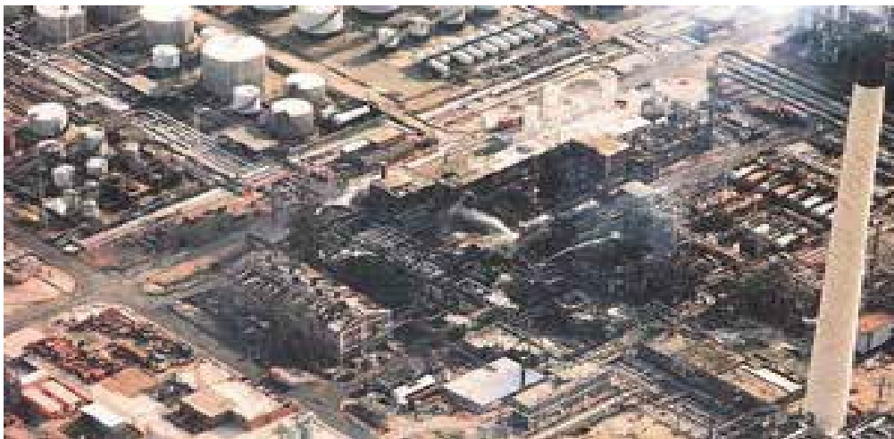
Figure 5.13 Aerial View of Ethylene Oxide Plant after Explosion
