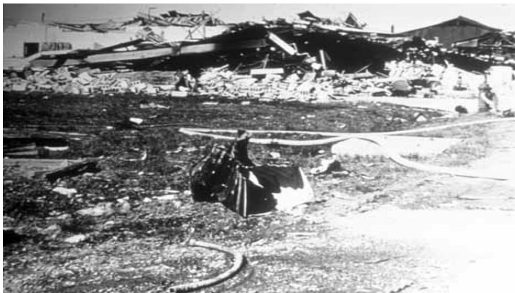
Figure 5.5 Plant Laboratory After EO Vapor Cloud Explosion, 300 Feet Away from Explosion Center
