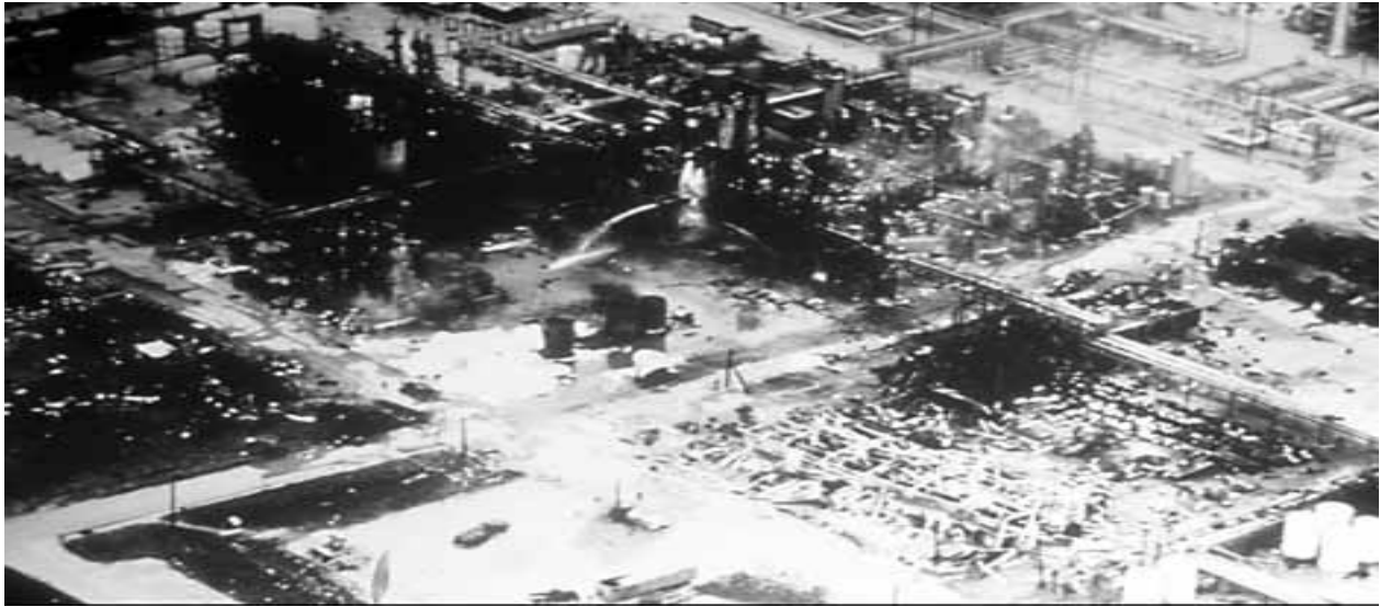
Figure 5.3 View of the Plant Showing Overall Damage
