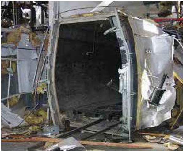
Figure 5.27 Damage to the building wall from impact of sterilizer door
