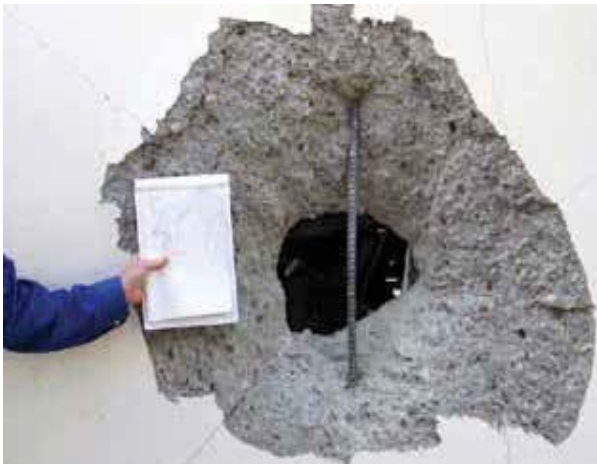
Figure 5.27 Damage to the building wall from impact of sterilizer door
