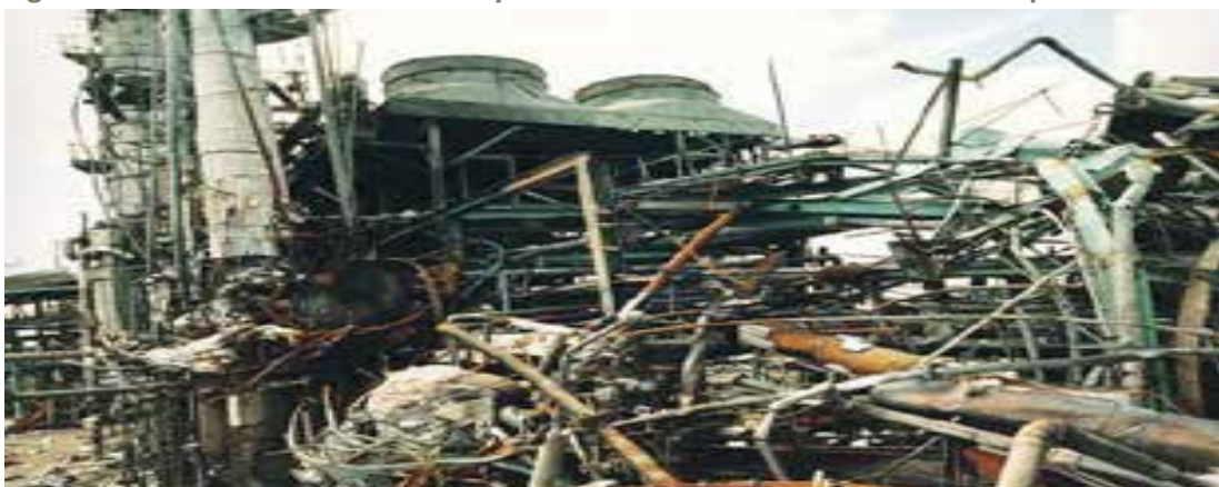
Figure 5.14 Remnants of Base of Ethylene Oxide Distillation Column after Explosion
