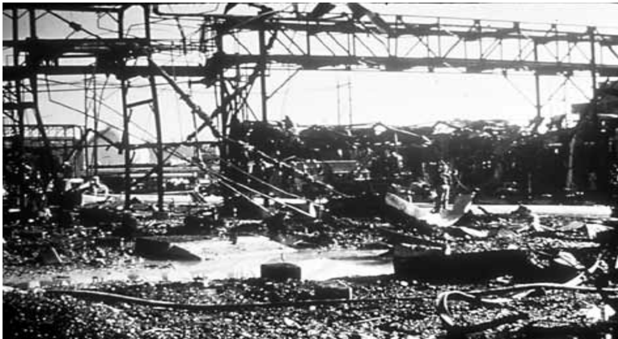
Figure 5.2 Blast Center after Explosion – EO Vessels No Longer Visible
