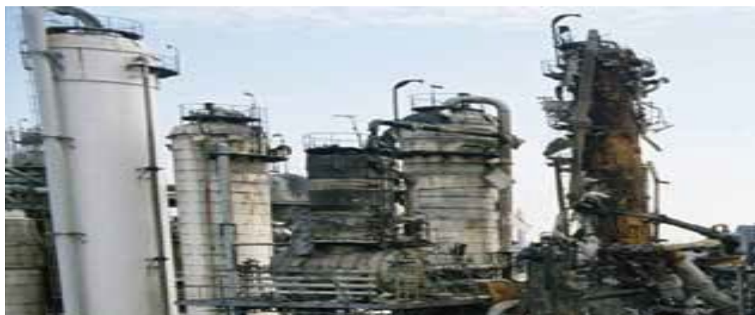
Figure 5.16 Aerial View of EO Unit After Explosion
